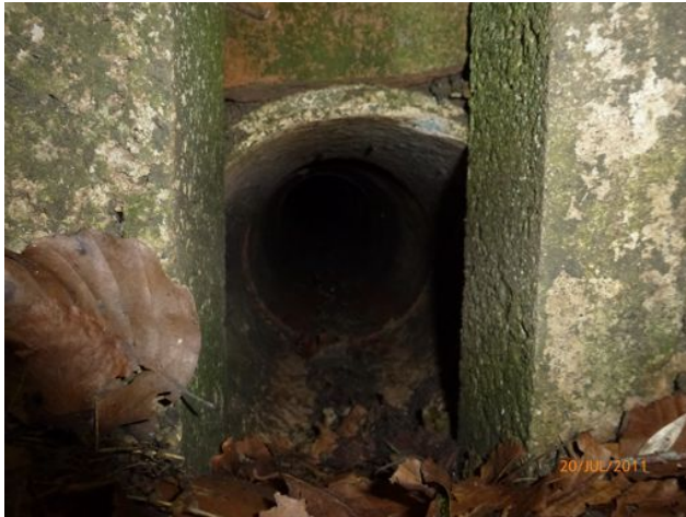
Fig 7: Ceramic pipes seen from the entrance of an artificial earth at Shrubs Coppice.
